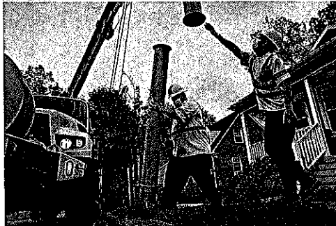
Workers put together pipe sections to drain a flooded catch basin in Alexandria, Va., in August 2021. (Michael S. Williamson/The Washington Post)
