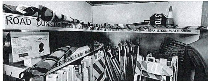
HBMWD Traffic Control Storage Room
