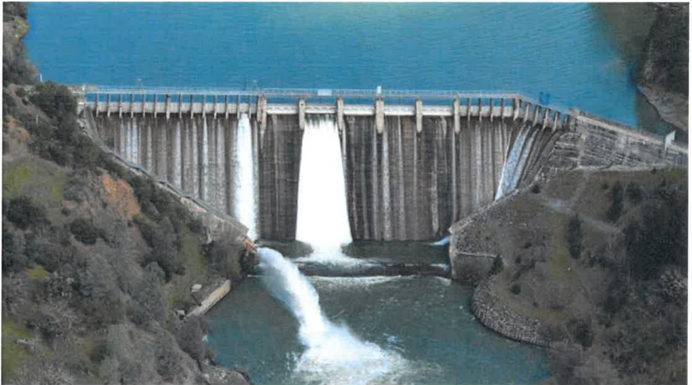
Scott Dam at Lake Pillsbury — a key component of the Potter Valley Project. | Photo courtesy PG&E.
