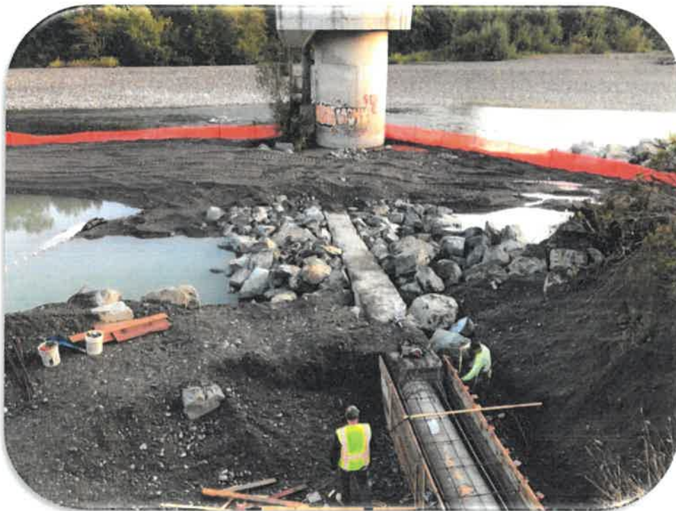
Collector 4 Emergency Repair Work due to Storm Damage
