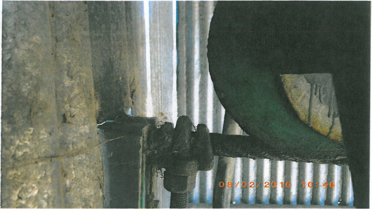
Photo 9 – Trolley #4 Rear Wheel
