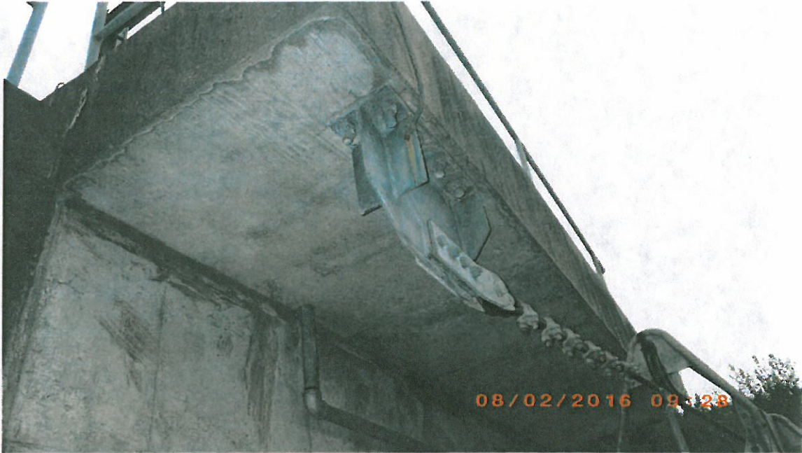
Photo 5 – Trolley #1 Cable Connection at Collector Well
