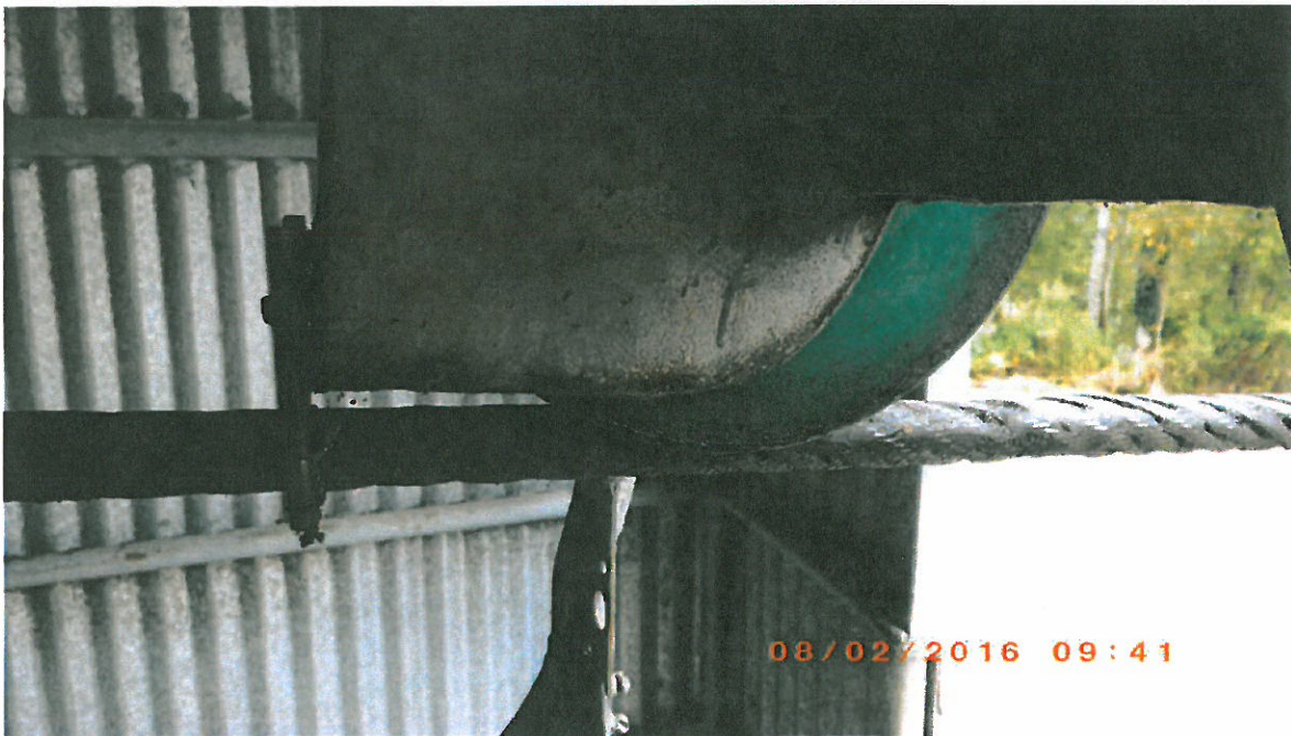
Photo 2 – Trolley #1 Rear Wheel
