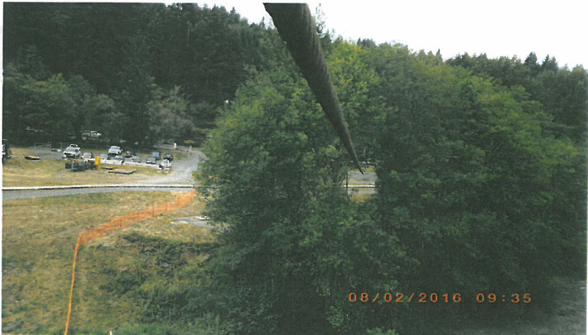
Photo 4 – Trolley #1 Cable Drape at Collector Looking Back
