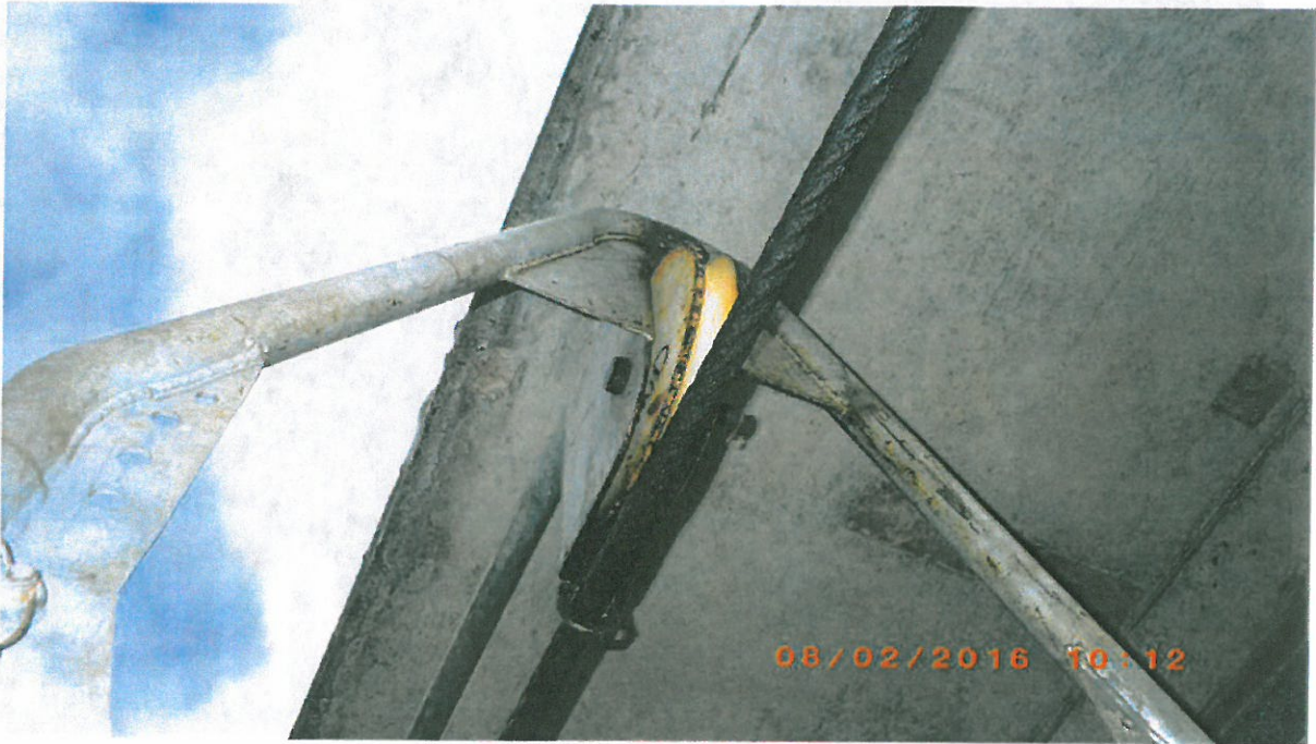
Photo 7 – Trolley #2 Rear Wheel
