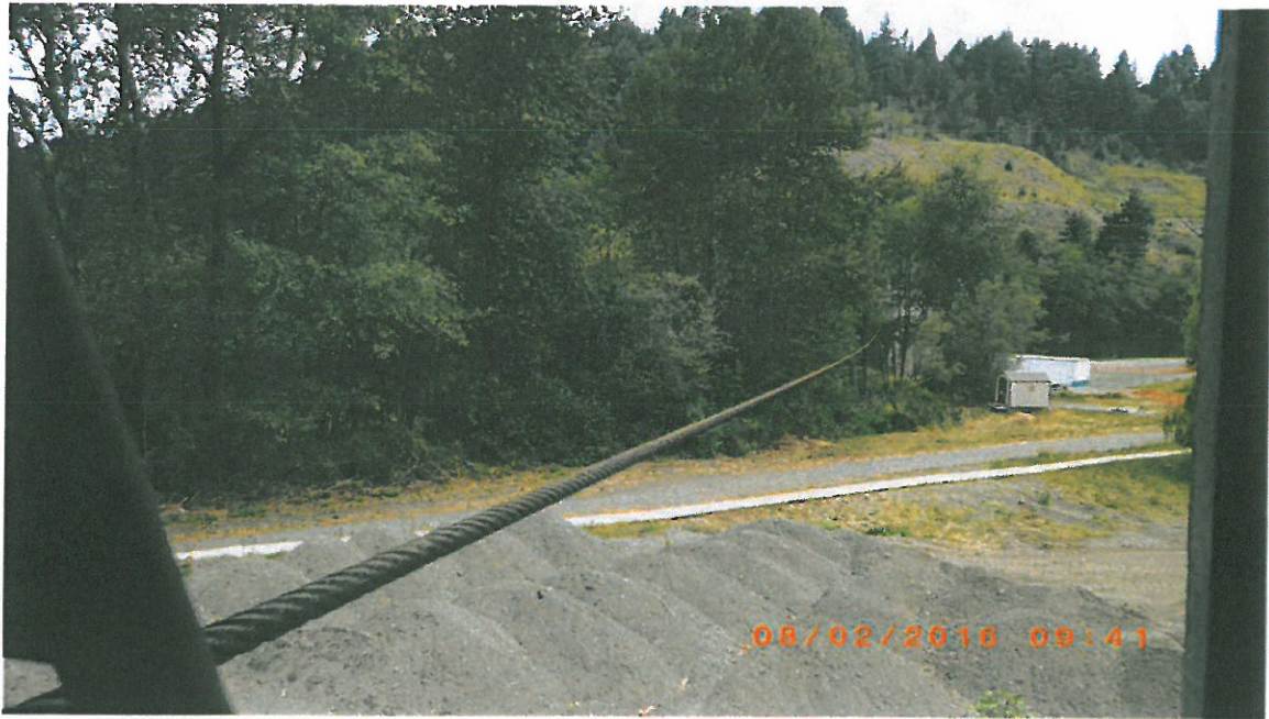
Photo 3 – Trolley #1 Cable Drape Exiting Trolley House
