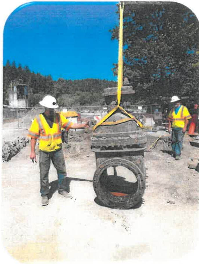
Collector 4 Valve Replacement
