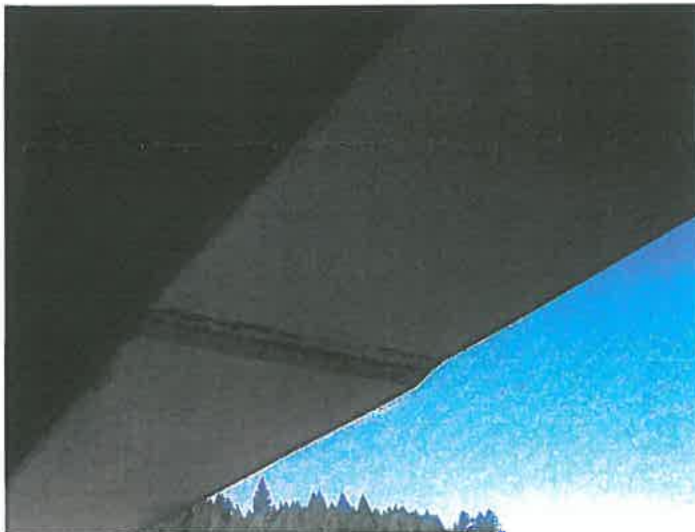
Photo No. 2 Butt welds at bottom flanges
