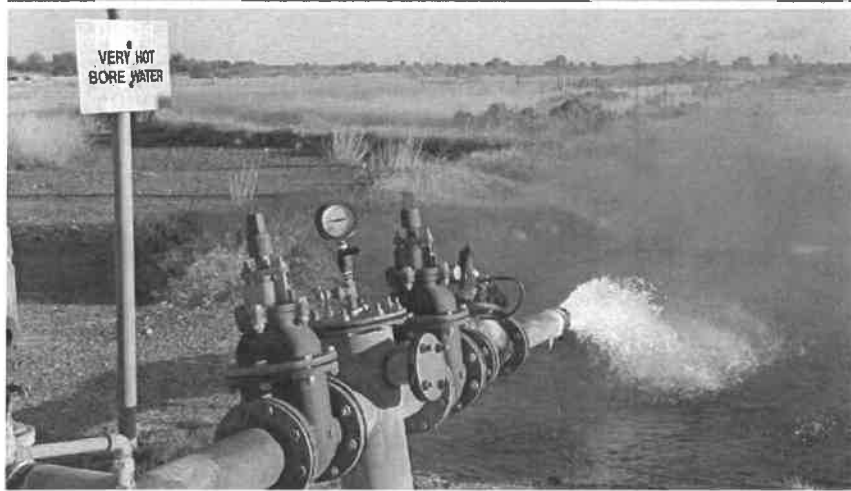
Groundwater being pumped from the Great Artesian Basin, Australia, to produce hydro-electric power. GETTY IMAGES
