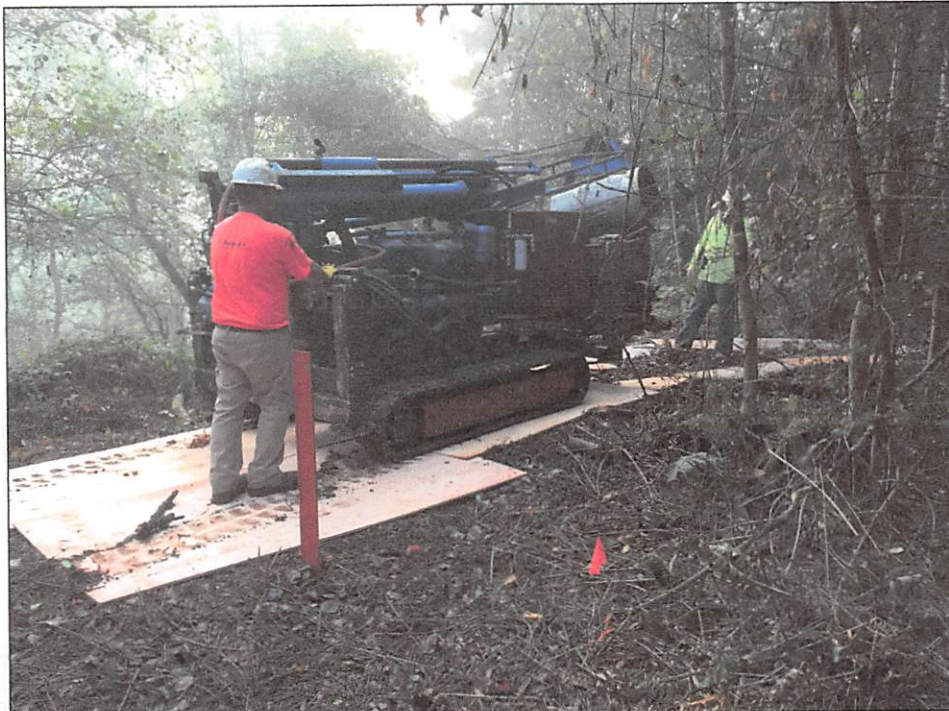
Photo 4. Walking drill rig on top of protective layer of plywood.
