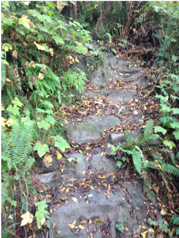
Picture 26: Steps cut in heavily weathered argillite along hiking trail downstream from the west bridge abutment.
