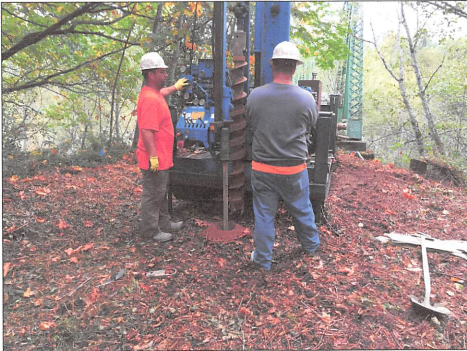
Photo 2. Coring at Test Hole 1.
