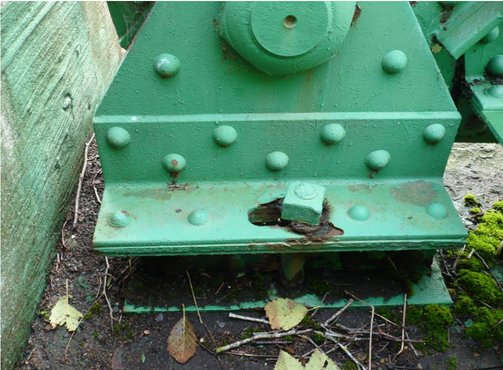
PIN ON PIER 1
