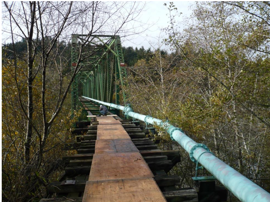
TRESTLE AT EAST END LOOKING WEST
