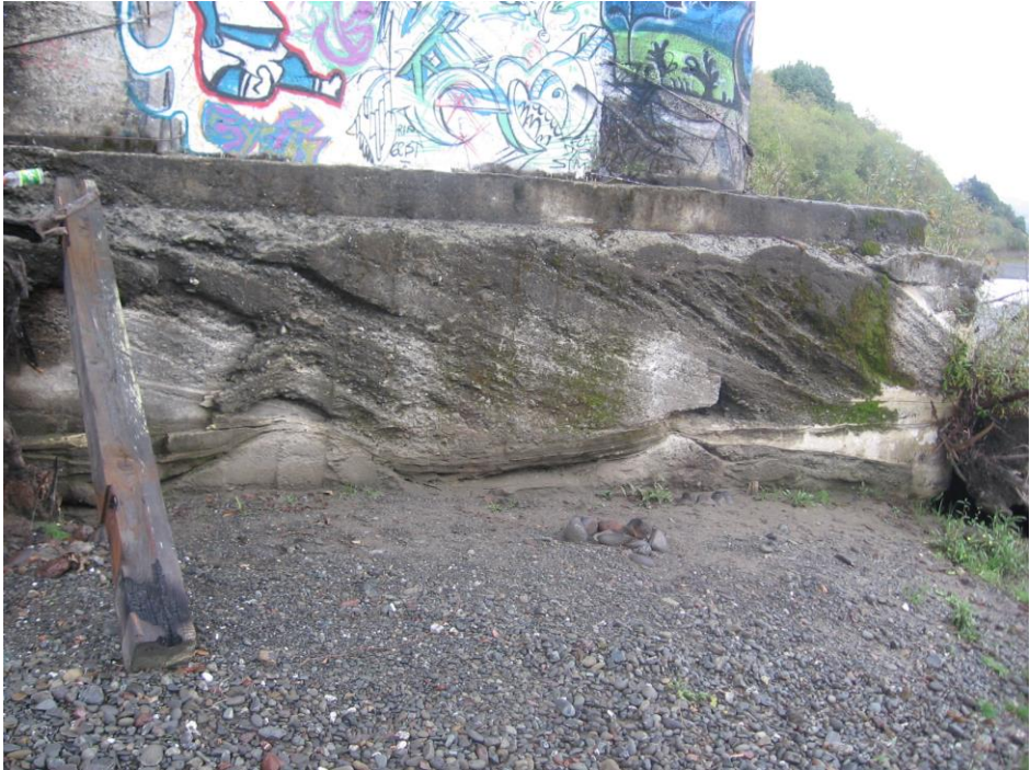
FOOTING PIER 3 FROM DOWNSTREAM LOOKING SOUTH
