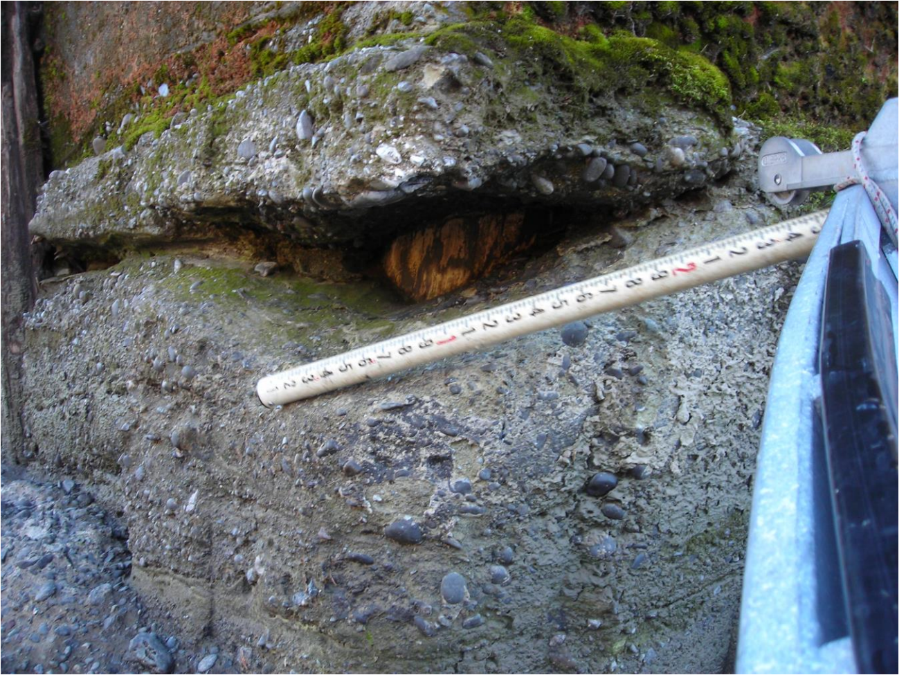
DETAIL OF EMBEDDED PILE ON NORTH END OF PIER 3
