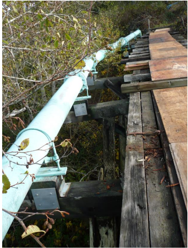
TRESTLE AT EAST END LOOKING EAST
