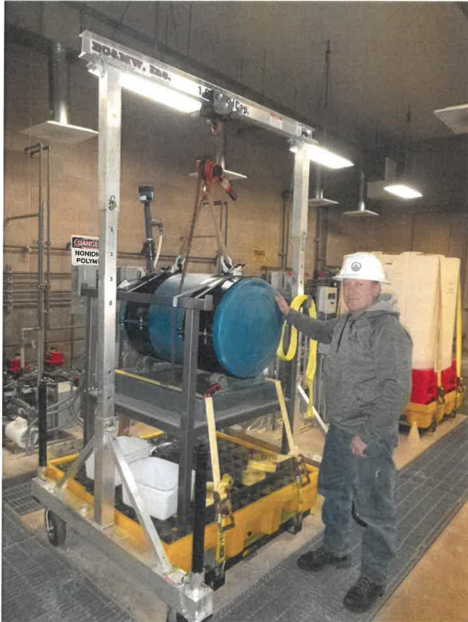
Working on water treatment plant chemical feed system.
