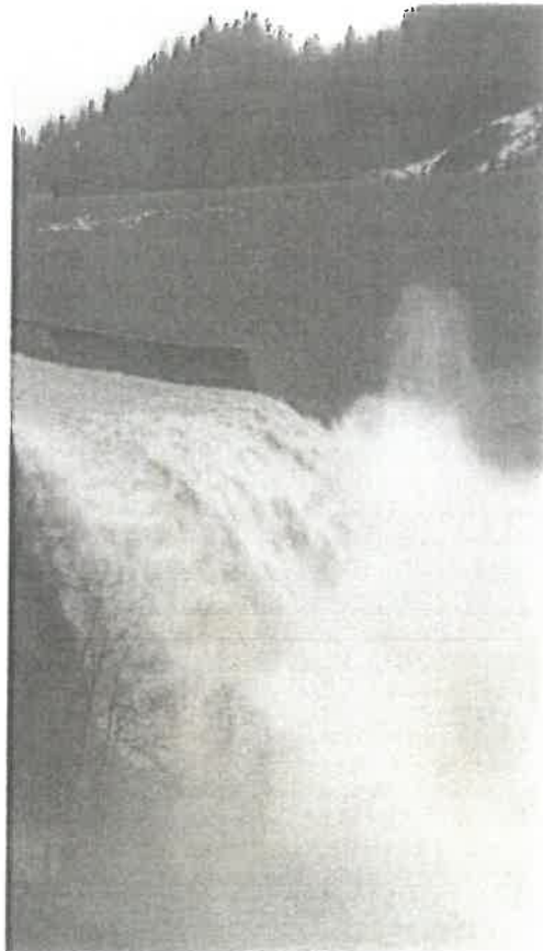
Ruth Lake Spillway 02-27-19
