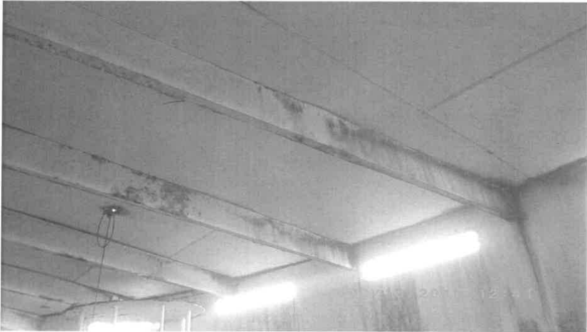
Photo 3 – Typical Air Vent at Interior Side
