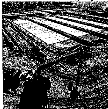
A new reservoir to capture rainwater.
