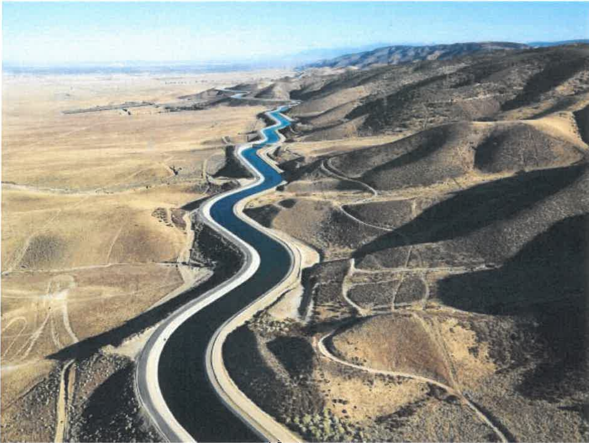
A portion of the California Aqueduct. Photo by iofoto, istock.com
