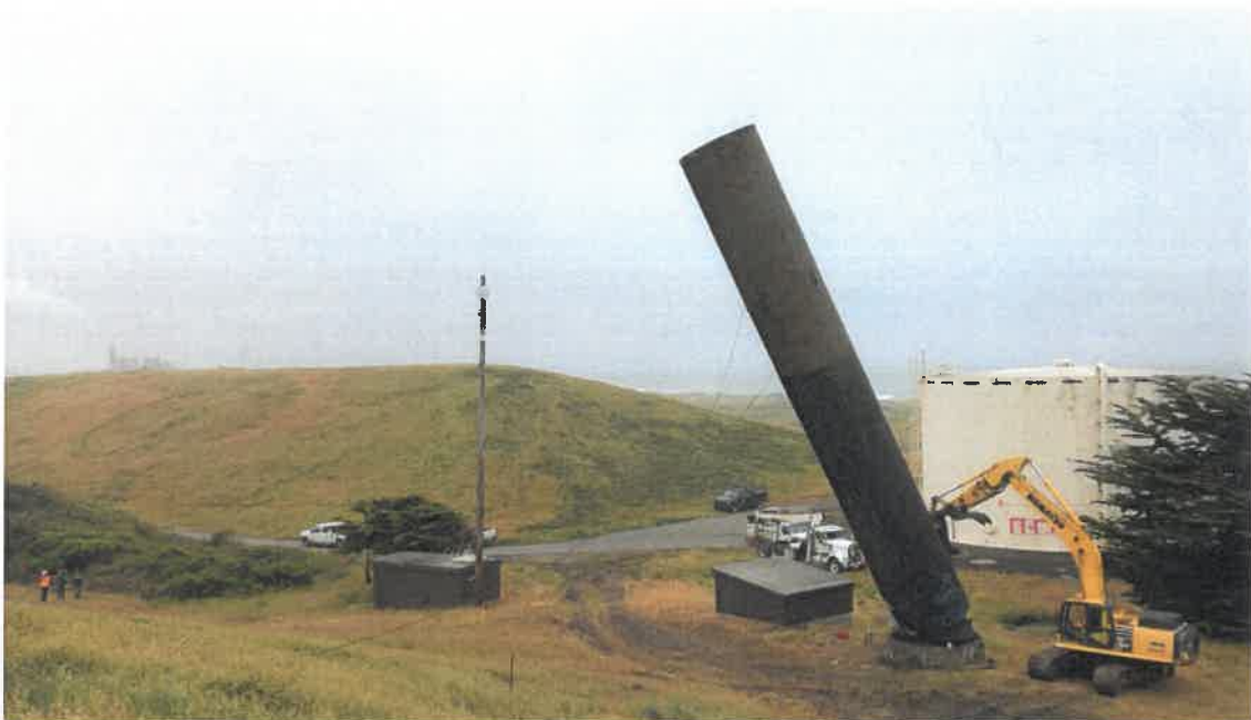
Surge Tower Coming Down
