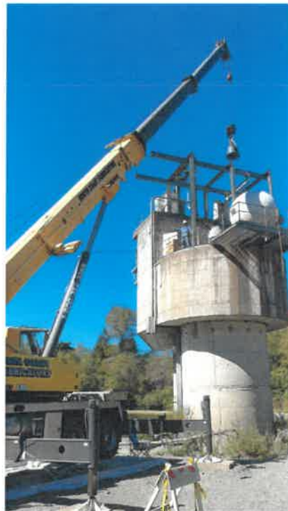
Pumps going in to Collector 1
