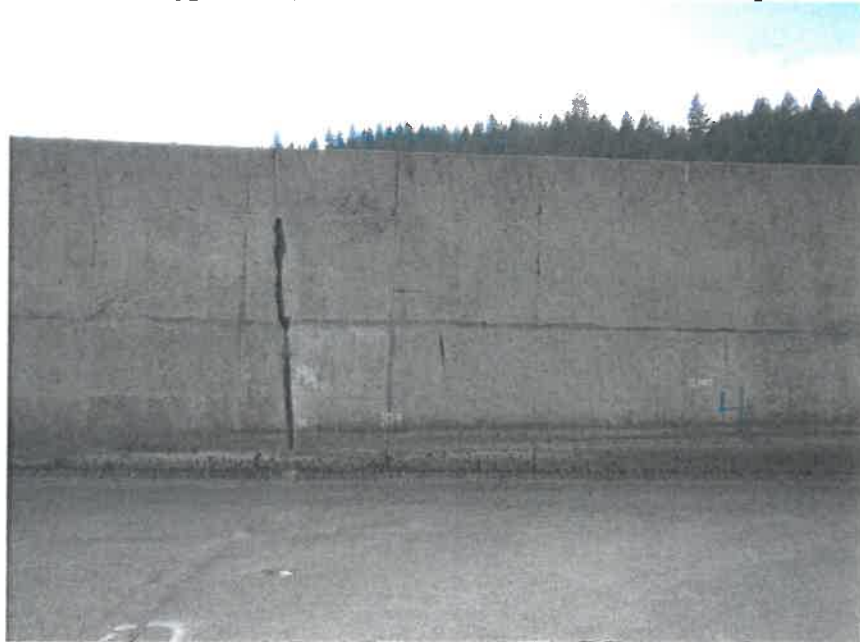
Photo #8 – Repair on downhill wall at joint between panels 4 and 5.
