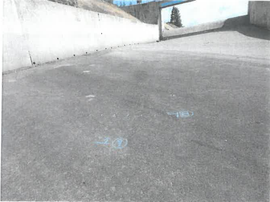
Photo #3 – Typical concrete surface of slab panel.
