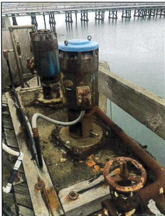
Image 2-14 RMT II-Existing Water Intake Pumps
