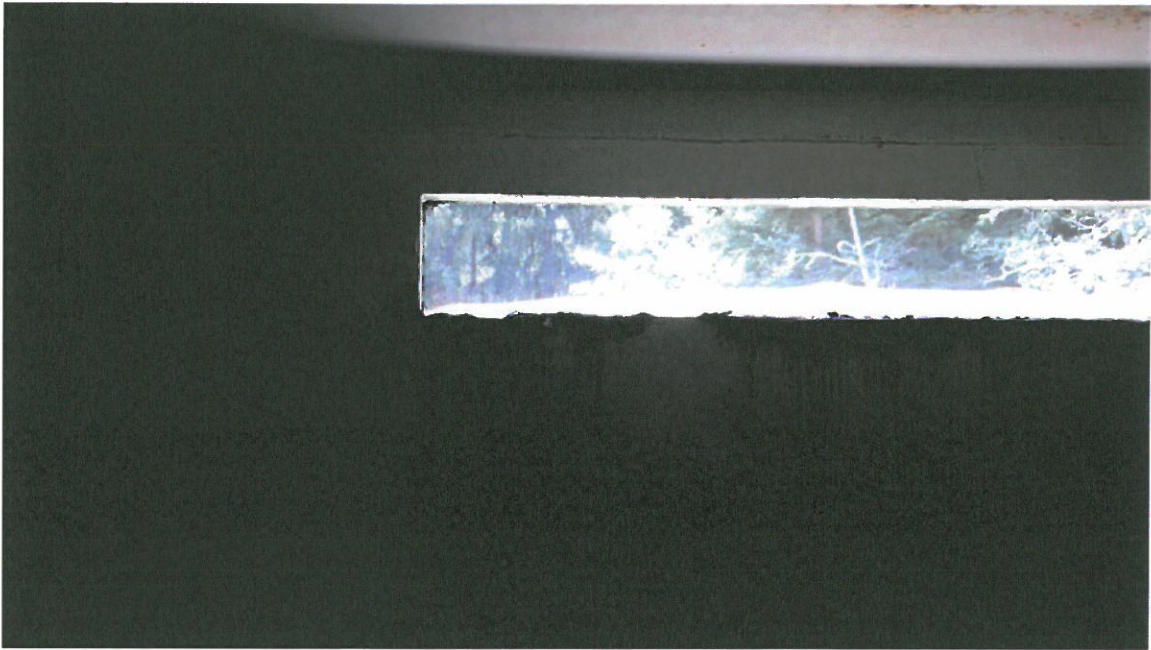
Photo 3 – Typical Air Vent at Interior Side
