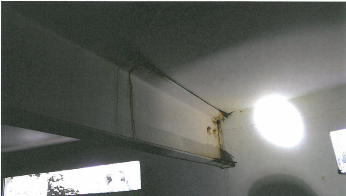
Photo 4 – Typical Channel Rafter at Perimeter
