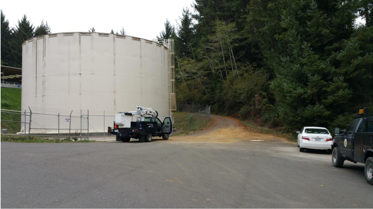
Photo 7: Tank Exterior (facing southwest)
