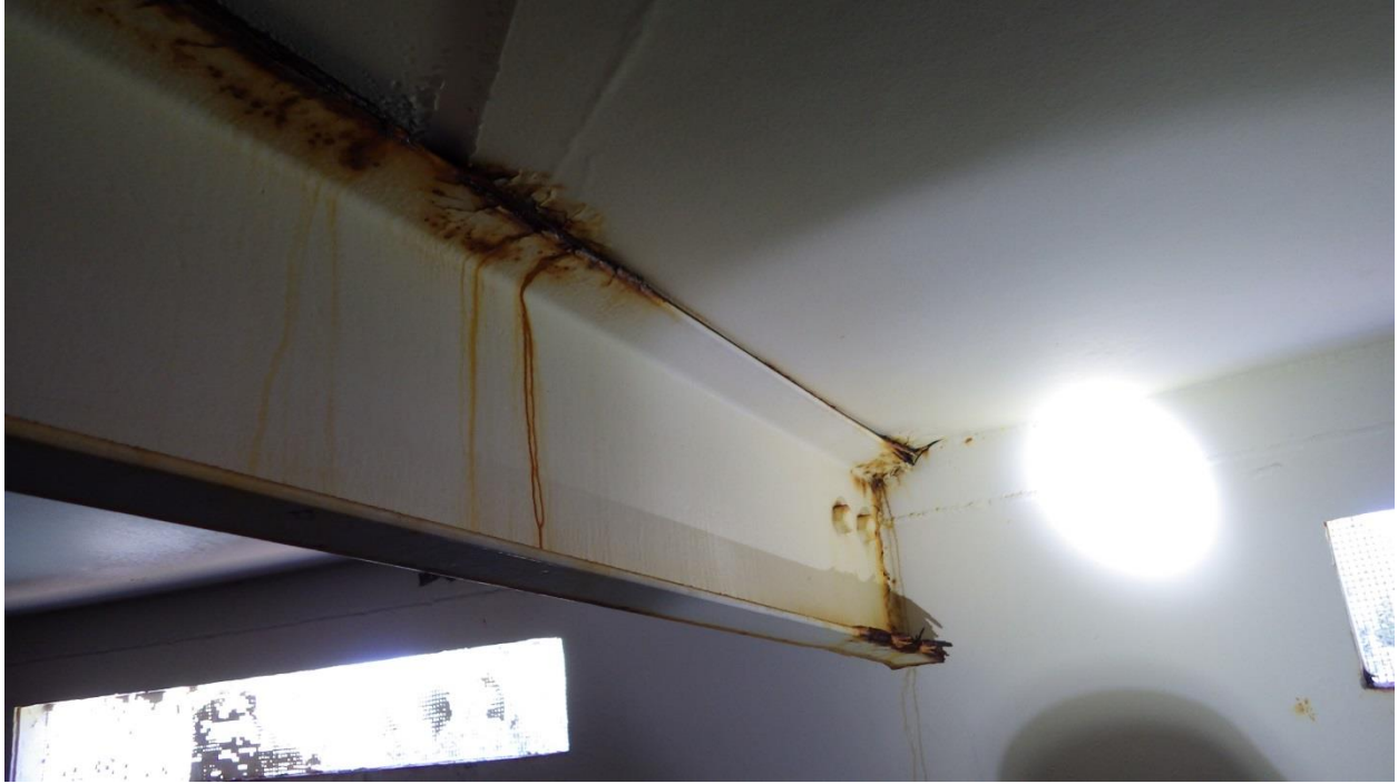
Photo 5: Typical Channel Rafter at Perimeter
