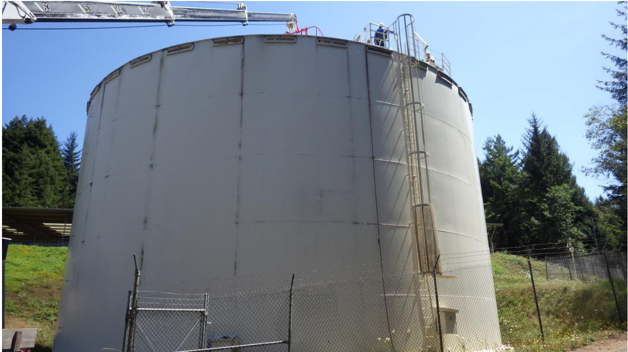
Photo 1: Tank Exterior (facing southeast)
