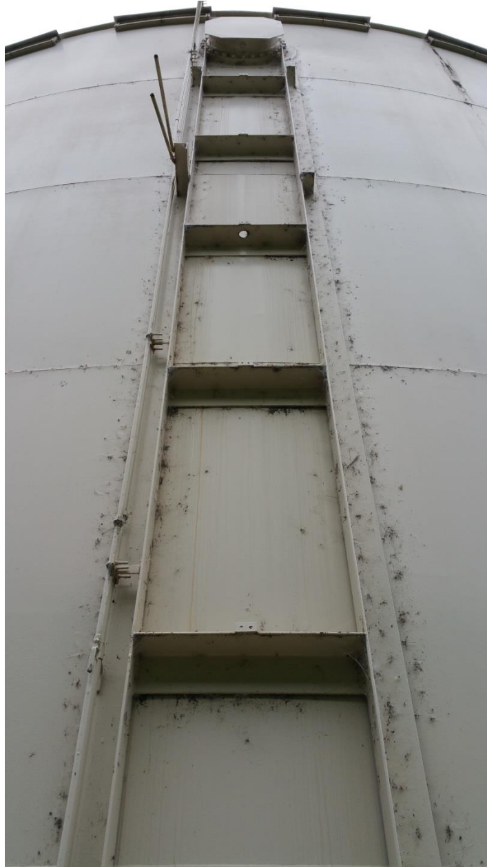
Photo 9: Former Inlet Pipe Support Structure
