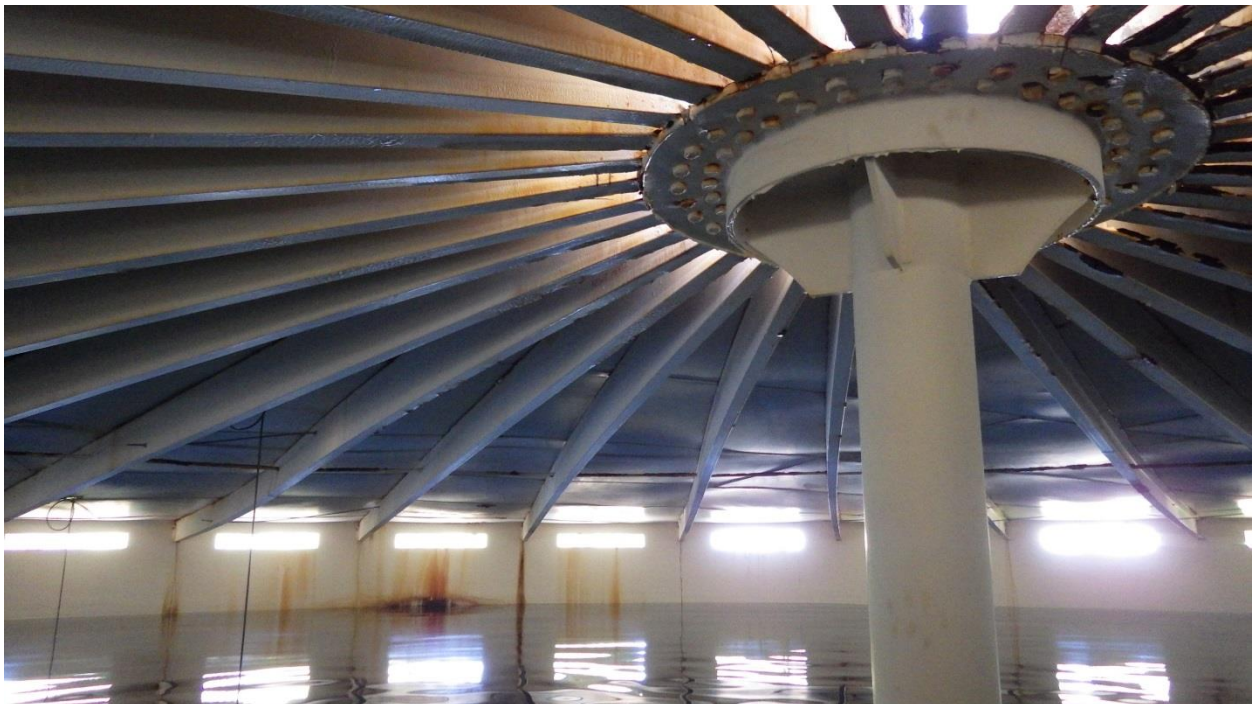
Photo 2: Tank Interior / Center Column Support
