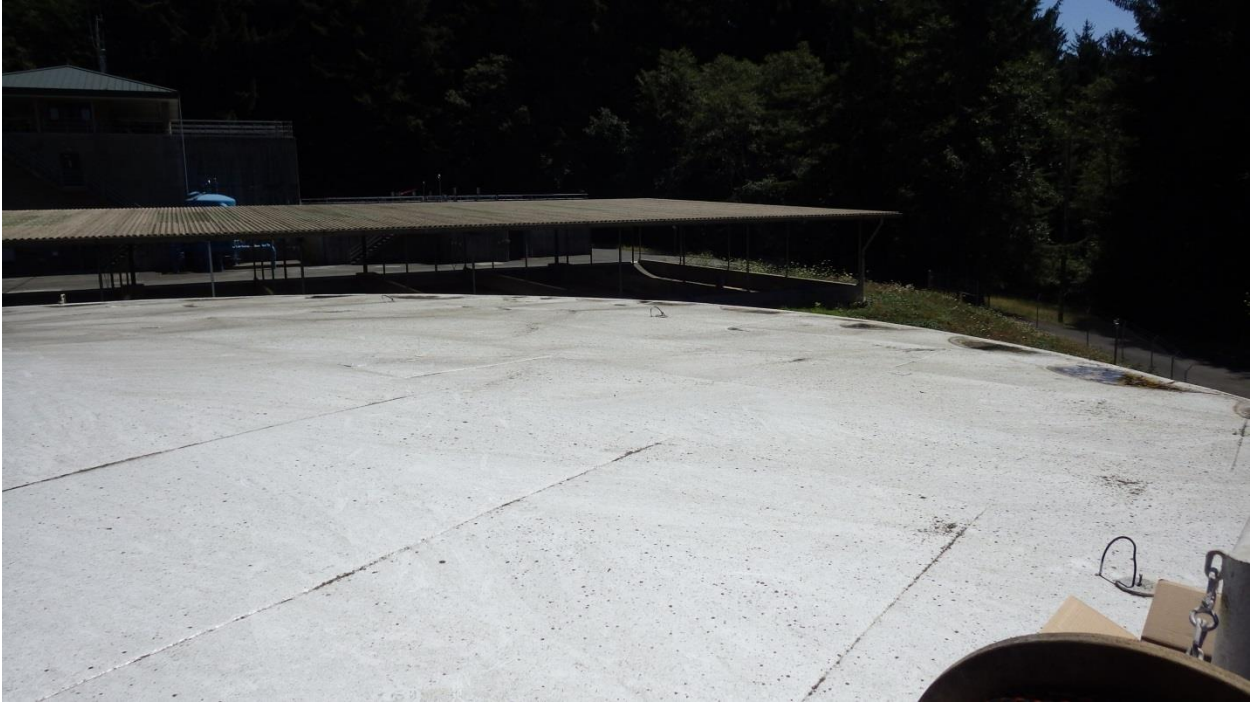
Photo 3: Exterior of Tank Roof
