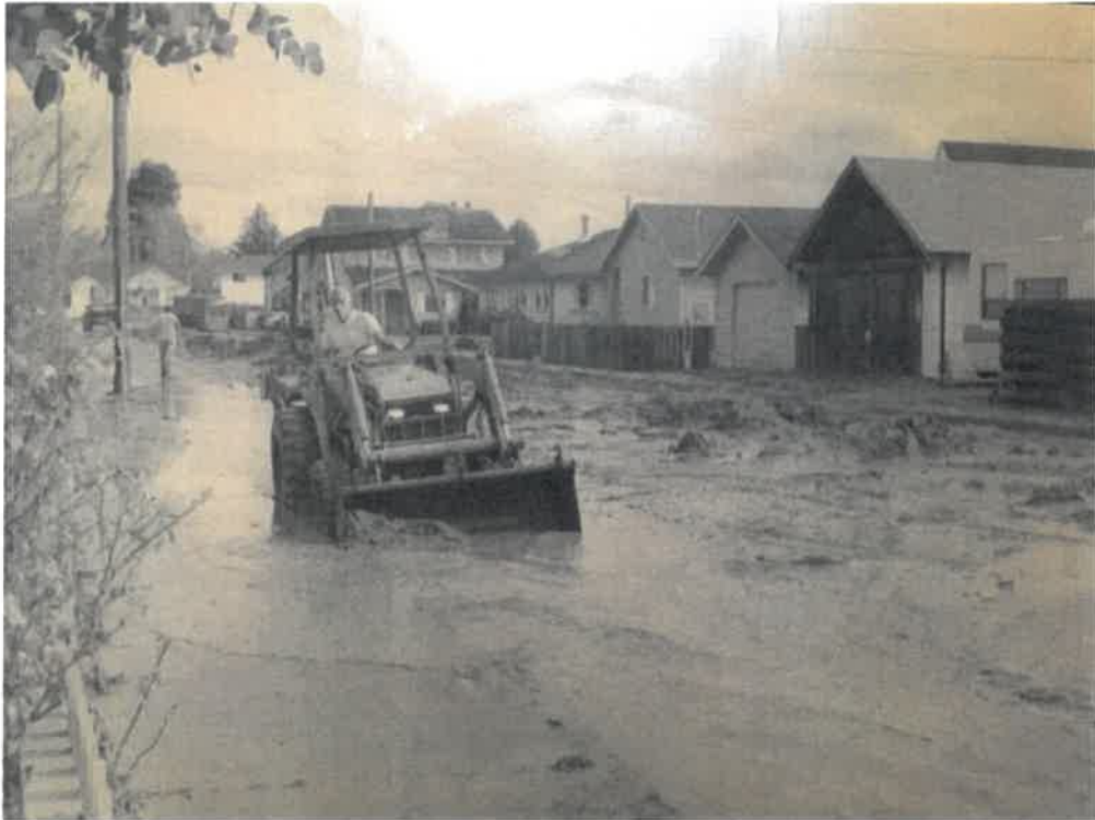
Henry Del Biaggio uses his own front loader to clear away mud covering A Street in Ferndale during the December 1996/January 1997 storms. (Times-Standard file photo)
