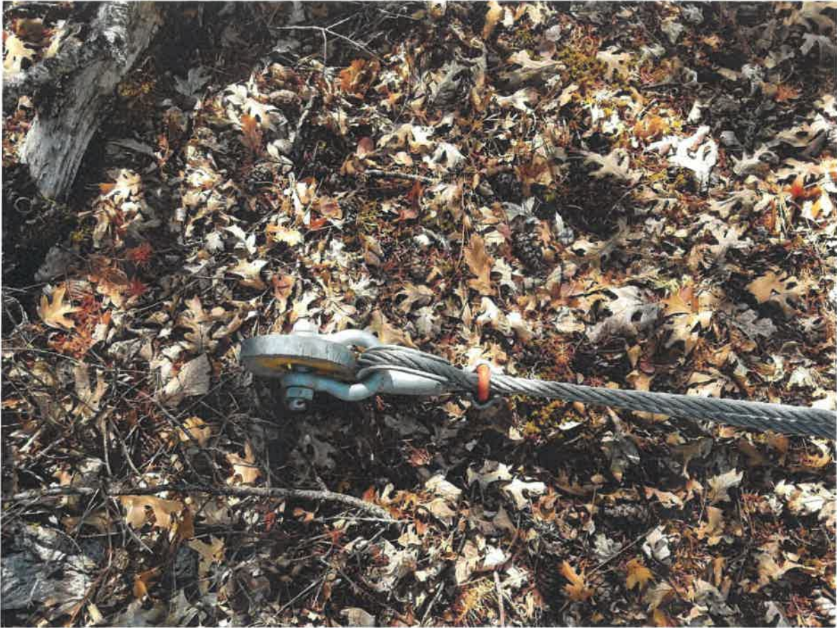
Photo 11-East End Anchor Connection
