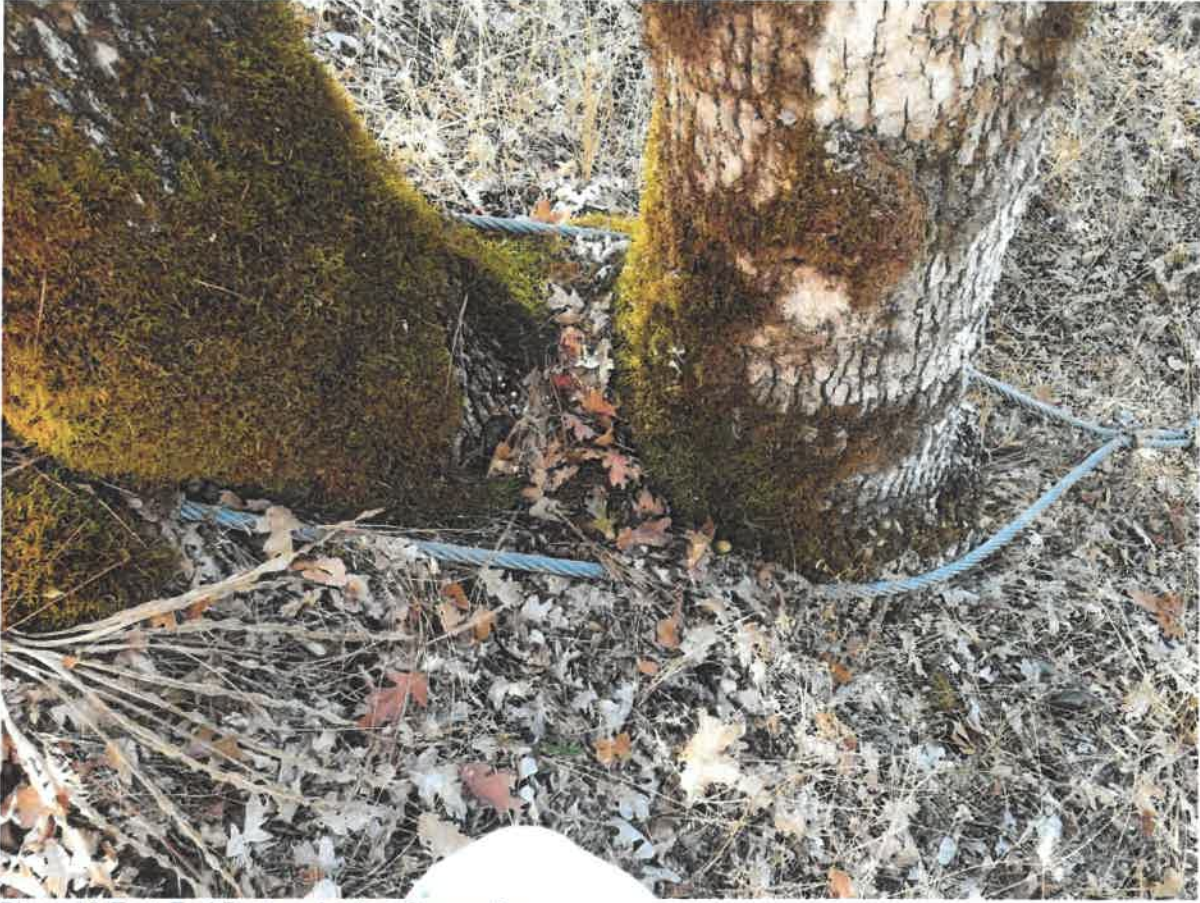
Photo 12-East End Backup Anchor Connection
