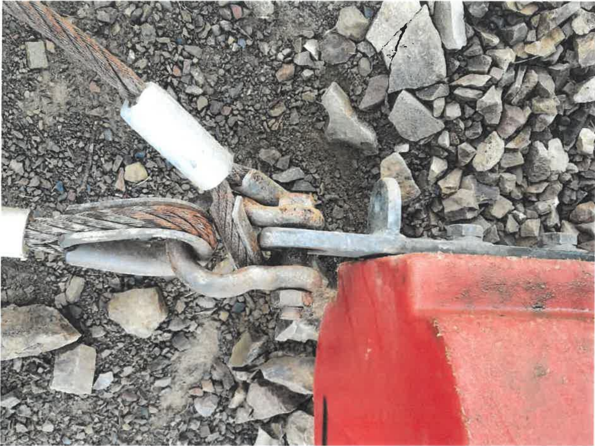
Photo 2-East Anchor Connection
