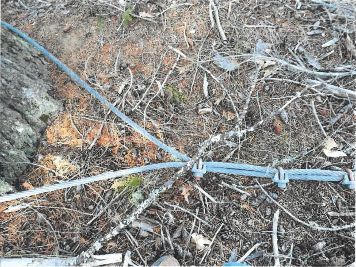
Photo 16-West End Back-up Anchor
