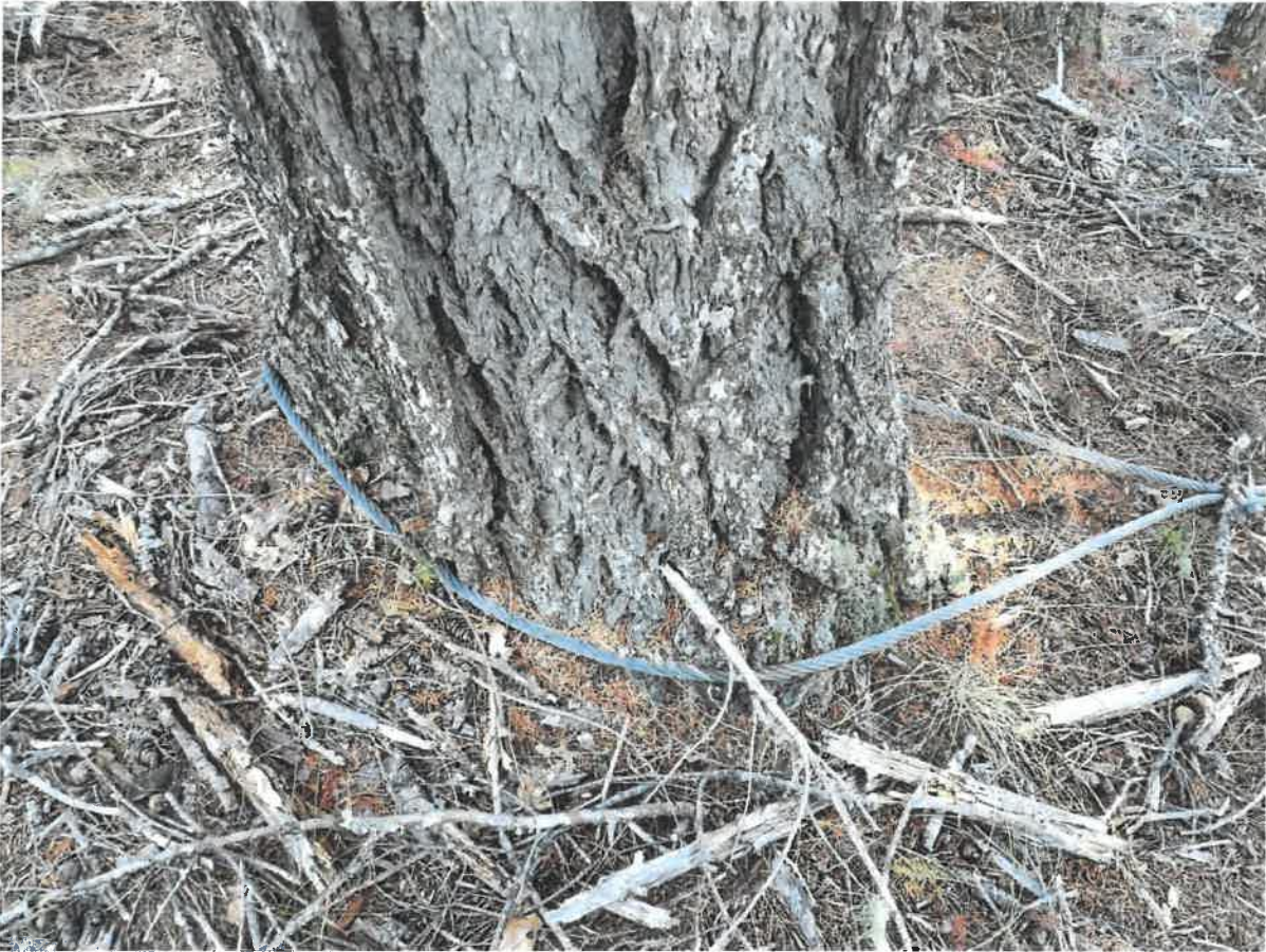
Photo 15-West End Back-up Anchor
