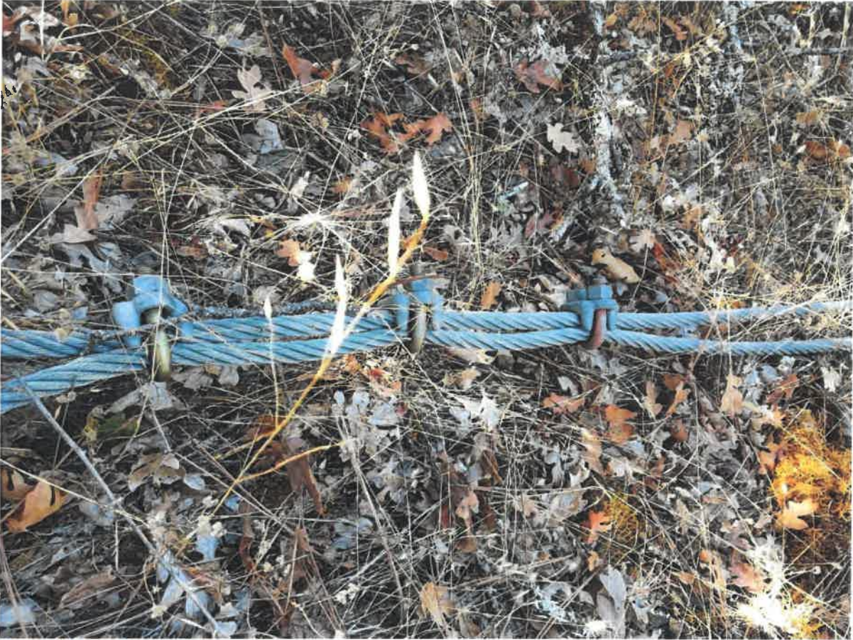
Photo 14-East End Anchor Cable
