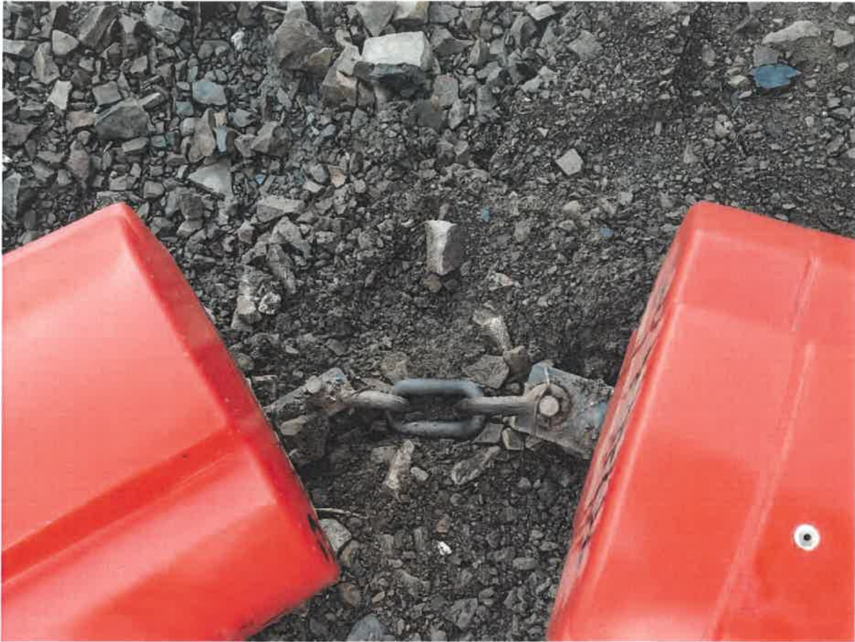
Photo 4-Connection btw Sections 1 & 2
