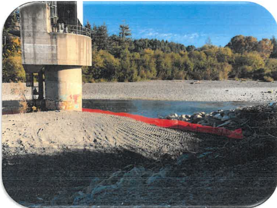
Collector 4 Completed Emergency Repair Work due to Storm Damage
