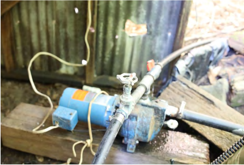
Water pump diverting water from a creek.
