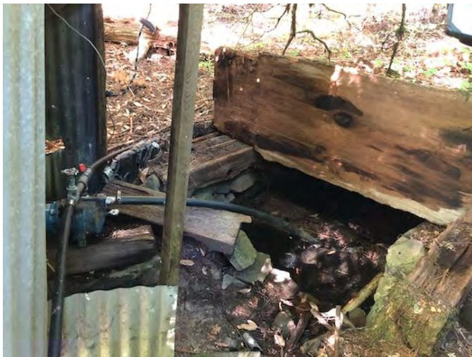
Active water diversion with pump.
