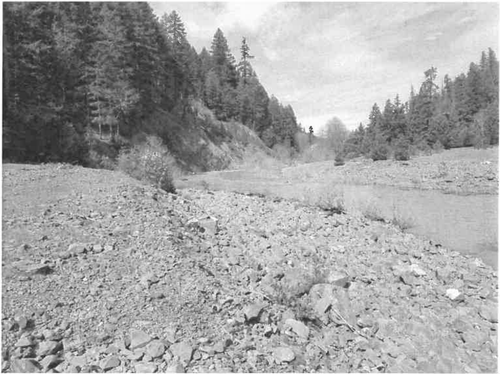
Figure 2: Downstream portion of project area. Flat for depositing sediment begins on left side of photo.
