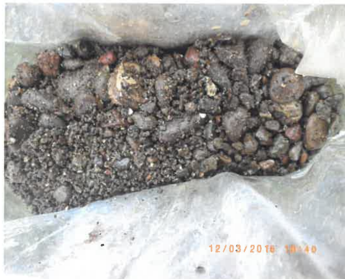
Figure 3: Rocks removed while installing projection pipes for new laterals
