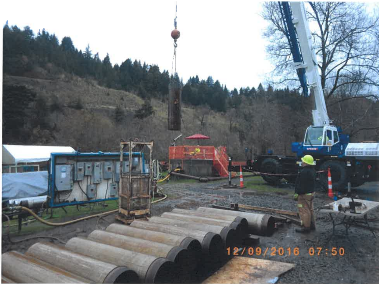
Figure 1: Projection pipe that the screened laterals were installed within
