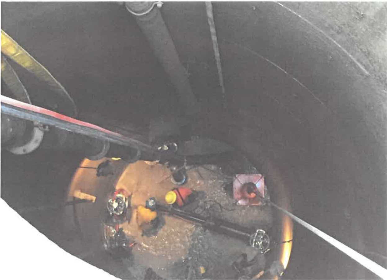
Figure 5: Installation of new laterals inside the caisson of collector
