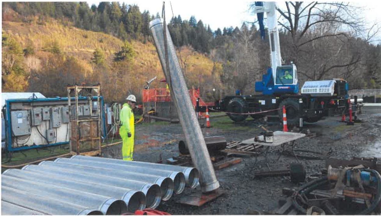
Figure 4: New screened laterals being lifted into caisson
