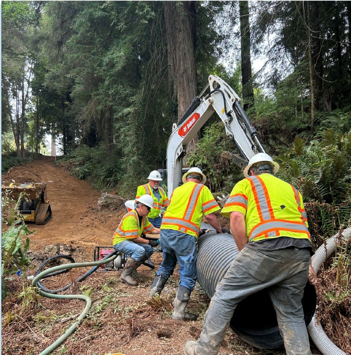
Figure 2: Emergency Pipeline Repair, August 2025
