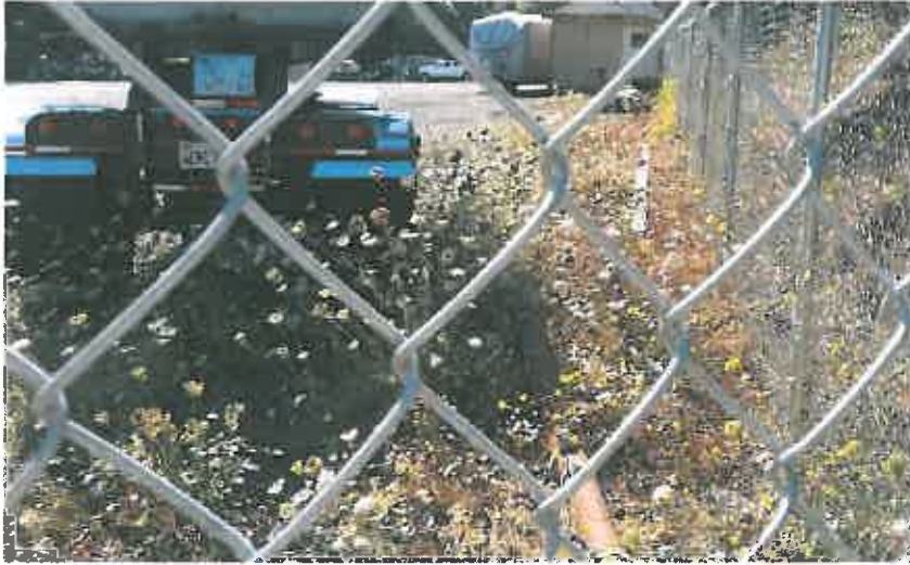
Photo 3. Eastern end of PSB on right bank (east side) of river
