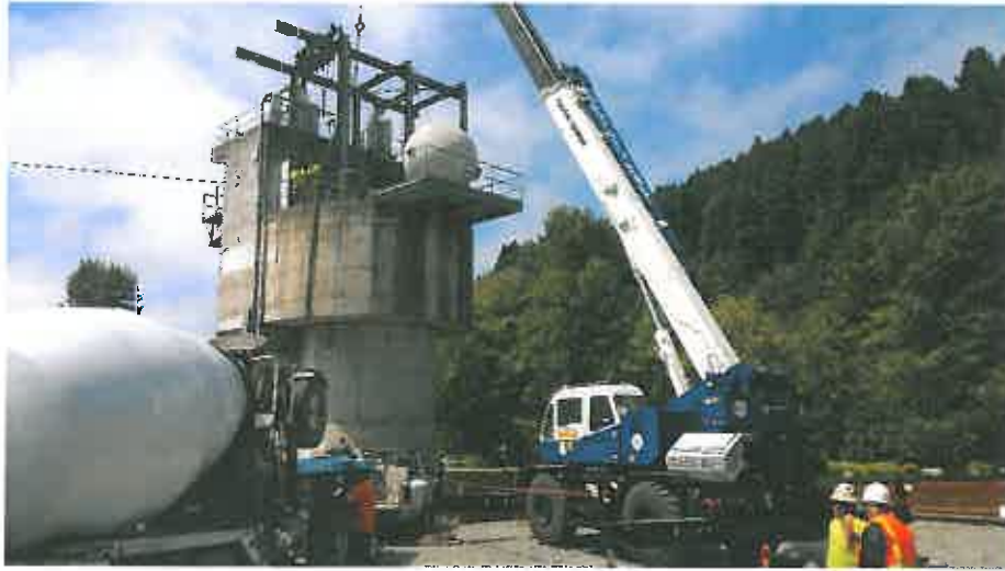
Ranney Collector 1 & 1A Lateral Project
