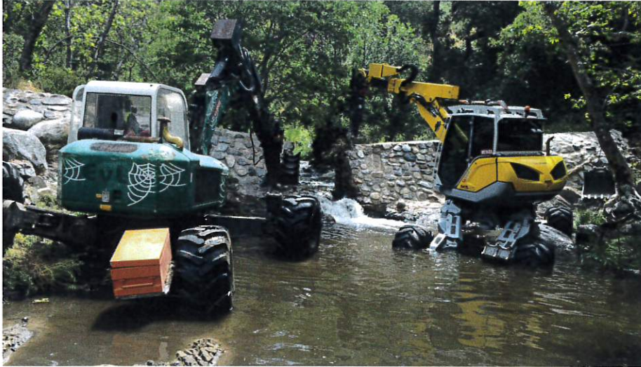
Spider excavators remove a dam on San Juan Creek in California's Cleveland National Forest. Photo: Julie Donnell, USFS
