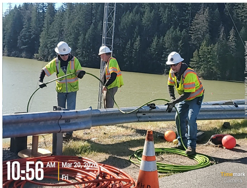
District staff handling hydraulic lines during operations, March 20, 2026.
