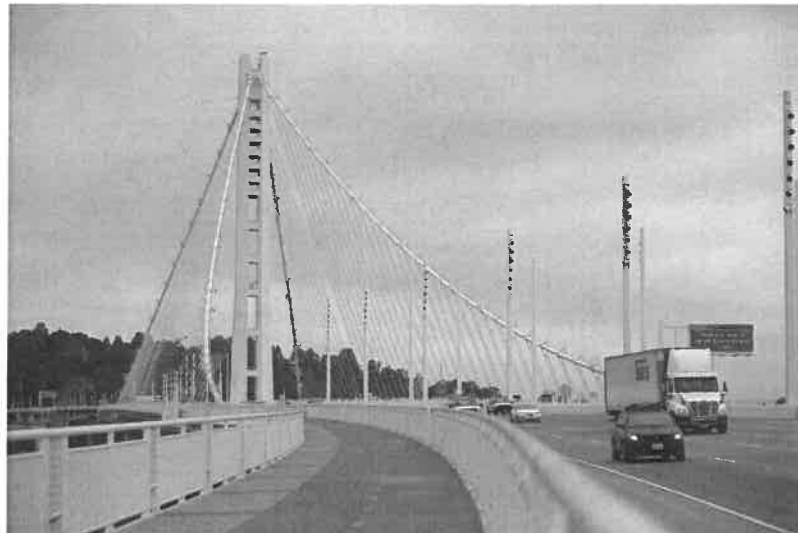
The Oakland-San Francisco Bay Bridge is designed to withstand earthquakes but remains vulnerable to storm surges. Justin/Sullivan/Getty Images
