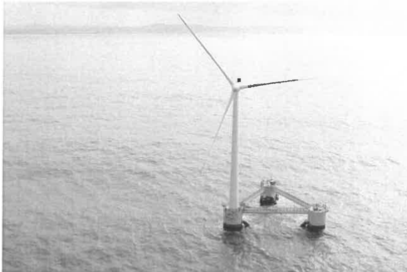
This floating turbine off Agucadoura, Portugal, is an example of the kind of energy generator that could be built off the California coast. MARC PREEL/AFP/Getty Images
