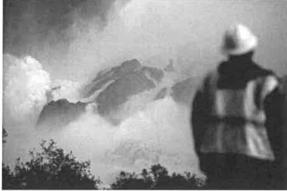
The Oroville Dam in California suffered damage to its spillway after intense rainfall. Josh Edelson/AFP/Getty Images
